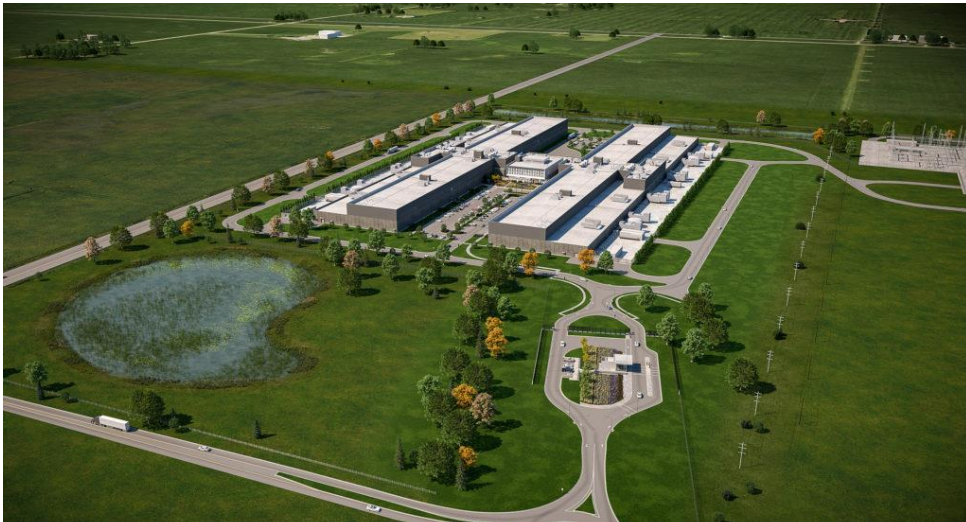
DeKalb data center that has been constructed
